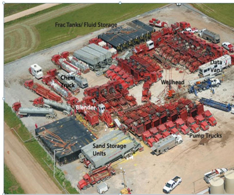
Figure 4: Aerial View of Typical Well Head Site Prepared for Hydraulic Fracturing 21
